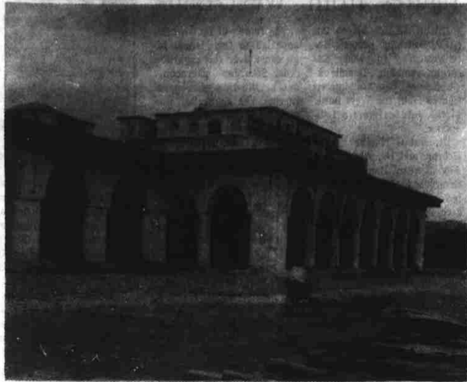
A view of Jahan Numa palace after completion of a part of its repair work.
